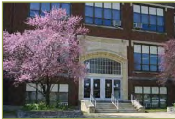
The front door to Lindenwood's new campus in Belleville, IL.
